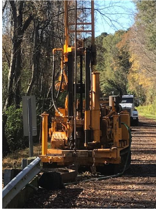
Drill rig on B-1
