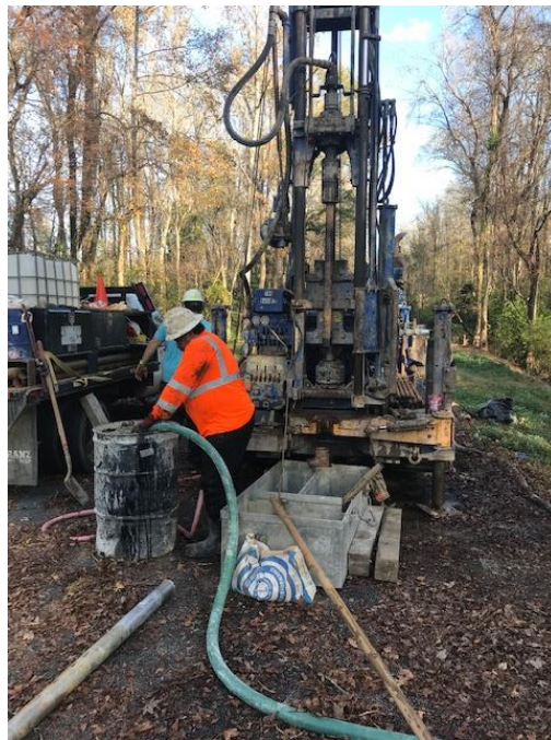
Drill rig on B-2
